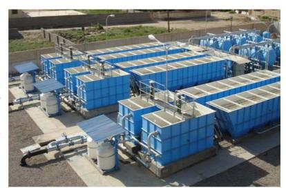
The chemical added water passes into sedimentation part and the flocks are settled down to the bottom of this tank. Treated water is stored in clean water tank and fed into the sand filters for final clarification.
