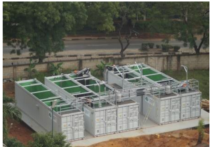
Containerized WWTP
